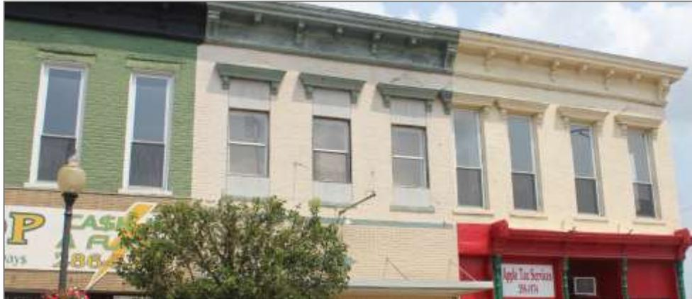
*Figure 4: The window openings on the center building were inappropriately reduced in size to accommodate replacement windows that do not match the original windows in shape, size, or material.*
