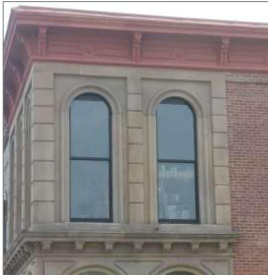
*Figure 3: The above image illustrates inappropriate window replacement as the windows do not match the original window shape or design and the replacement windows are vinyl clad.*
